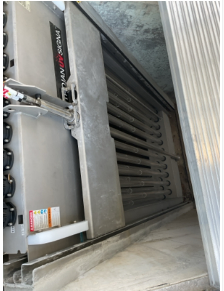
Bulb sleeves of the new UV
