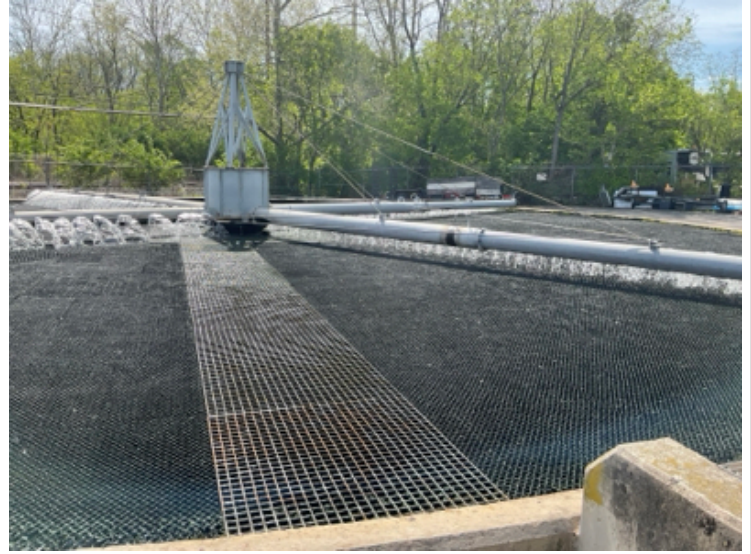
Second stage trickling filter
