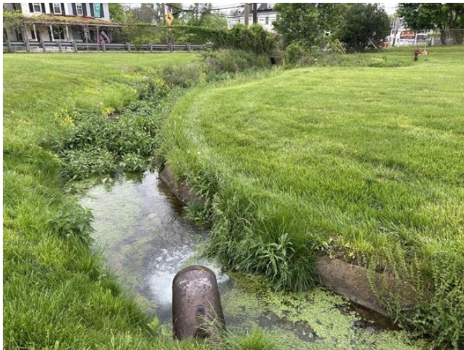
Pump spring house discharge outfall 004 and downstream
