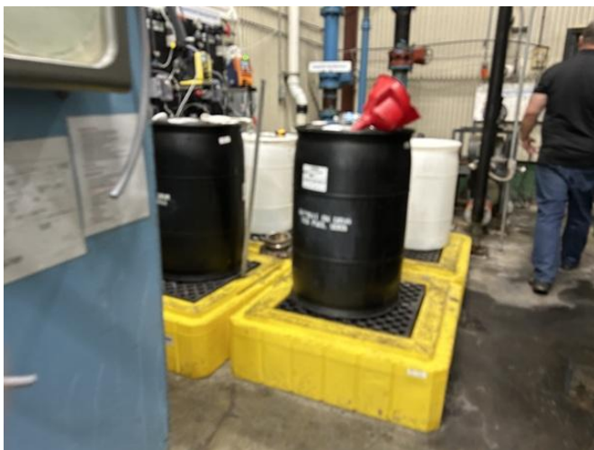
Operations building chemicals in containment
