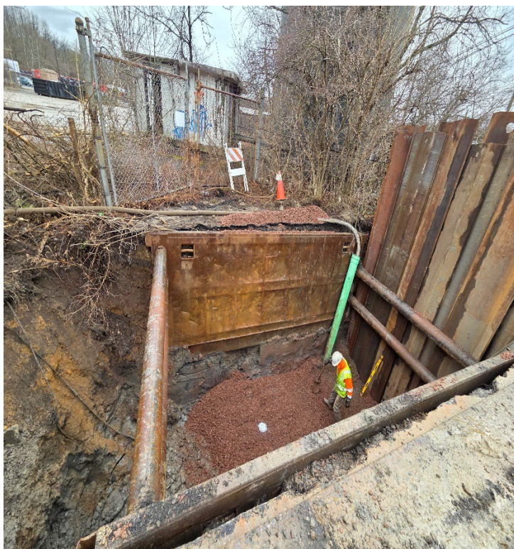
Launching Pit and Hydraulic Ram Machine
