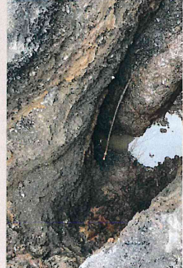
Maple Street replaced service line
