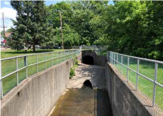
West of Reiff's Mill Road, Rose Valley Creek is channelized into a concrete flood control structure.
