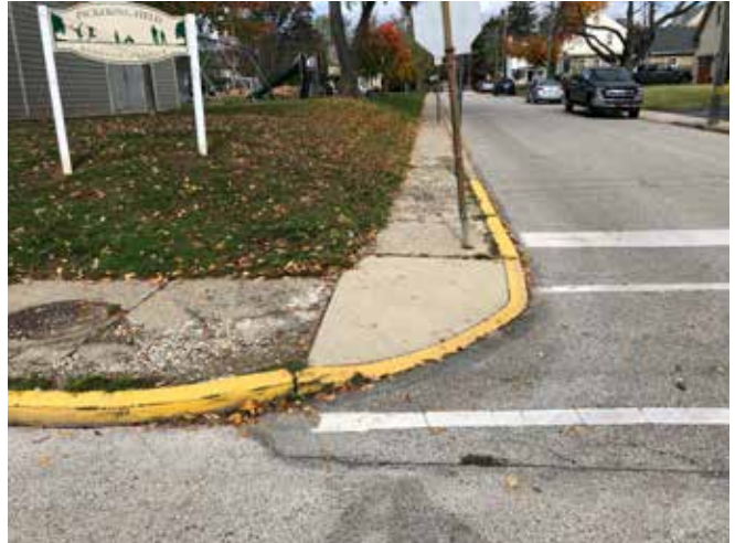
A curb ramp and poor-condition sidewalks at Highland Avenue and North Street.
