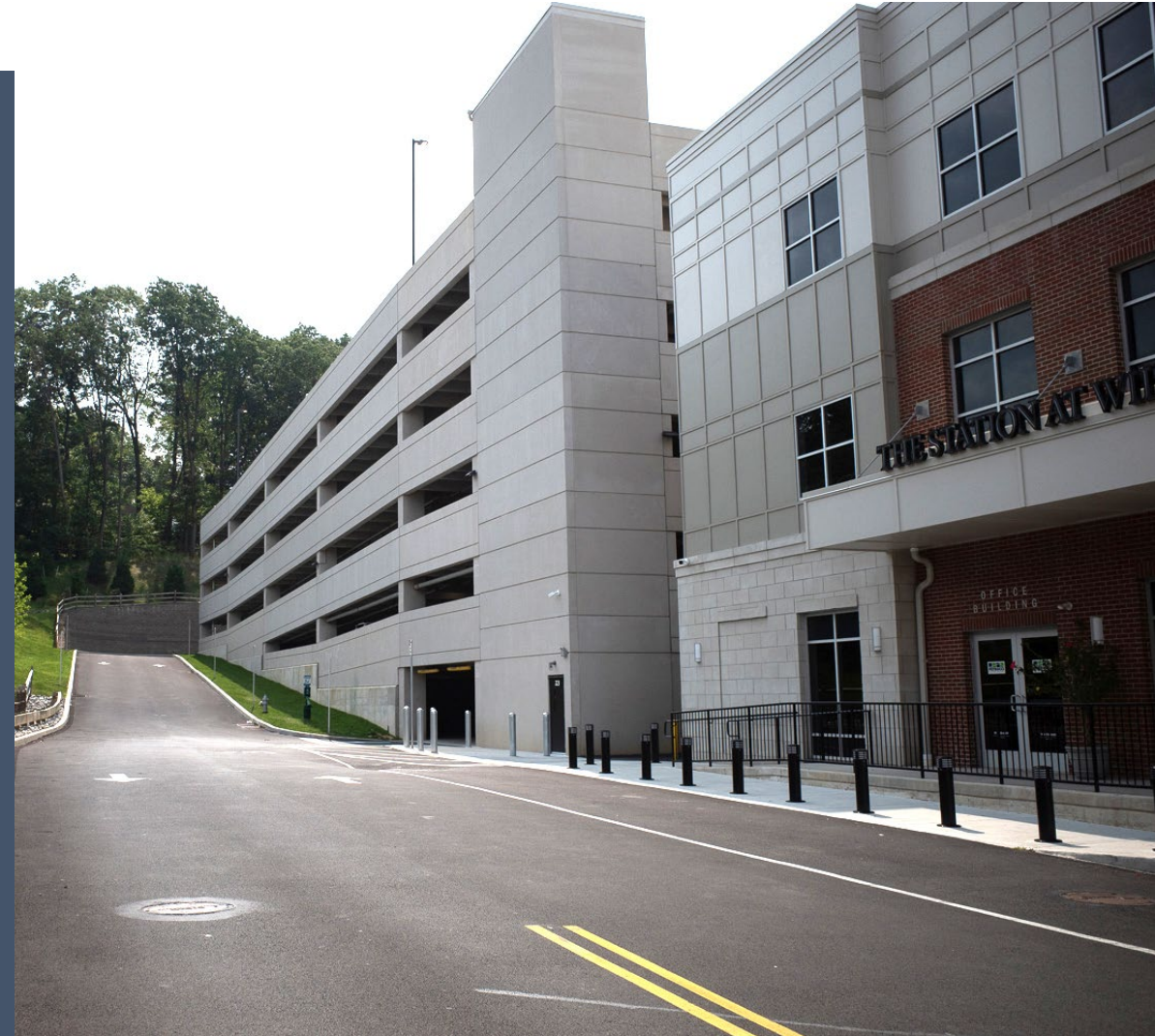
Rear parking garage accessible via alley
